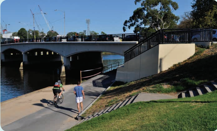
E-Crete used for new work on the Swan Street Bridge, Melbourne (Photo: Zeobond)
